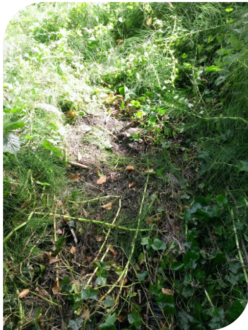
Photo 6— Upslope of inlet pipe with vegetation cleared. Note lack of channel.
