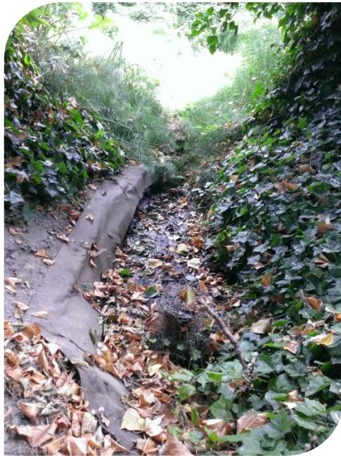
Photo 3— Concrete pond at toe of hillside. Screened, perched outlet in foreground.
